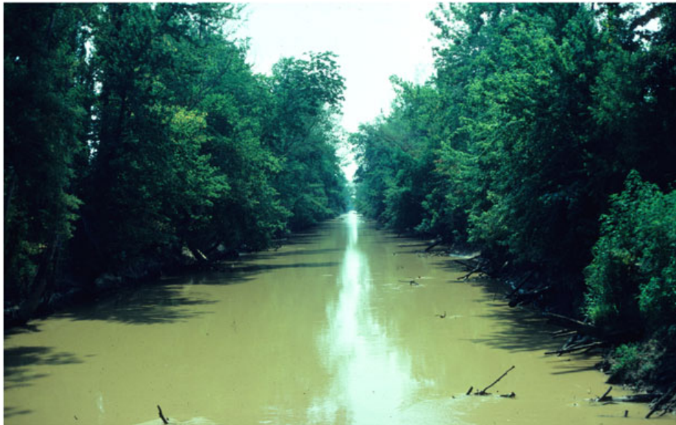
Figure 11. Photograph of the straightened channel of Obion River, western Tennessee. The channel straightening caused increased energy conditions and erosion despite abundant riparian-zone vegetation (photograph by W.R. Osterkamp, 1987). This figure is available in colour online at wileyonlinelibrary.com/journal/espl
