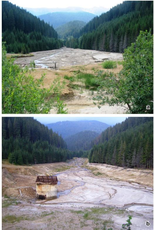
Fig. 2. Dumitreleul sediment retention reservoir, before sediment excavation in 2007 (a) and after excavation works carried out in 2009 (b) (figures from Pop *et al.* 2013).
